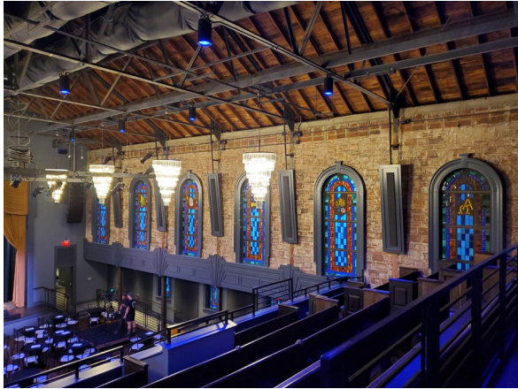
View of Auditorium from Balcony
